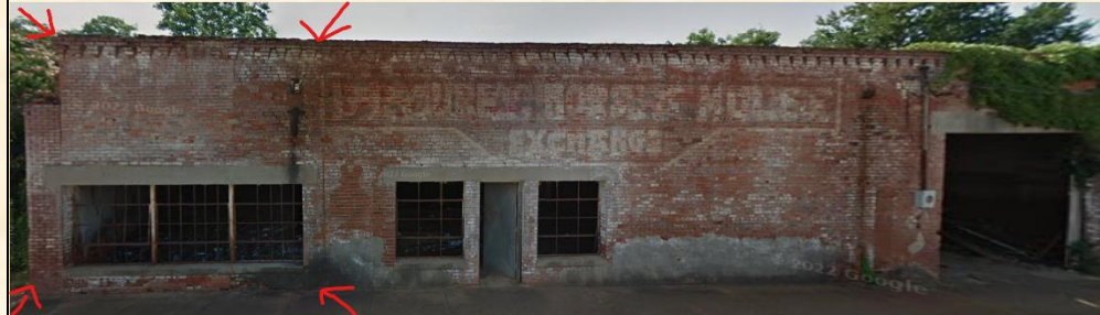
Northern portion: W R Curry Brick Store
