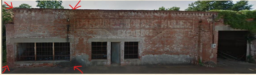
Northern portion: W R Curry Brick Store
